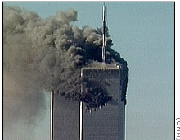
Fig. 9 North Tower After Impact Viewed From the Impact Side (Photo from CNN)
