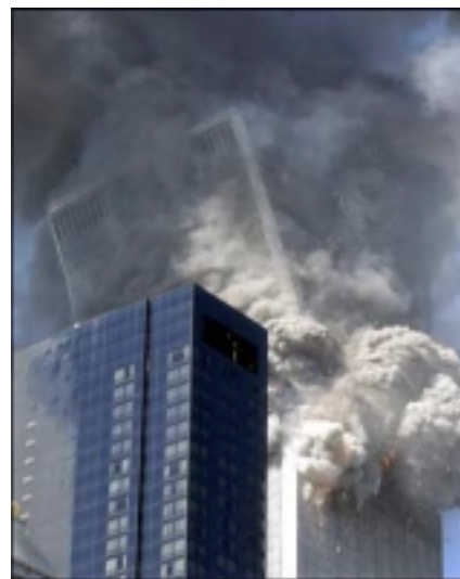
Fig.12 Top of South Tower Collapsing (Photo from CNN)
